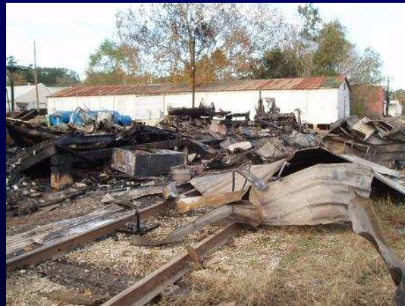
Gasoline storage facility
