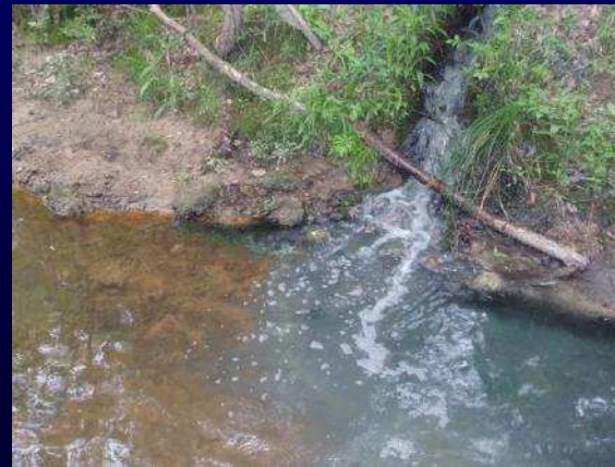
Sewer main break
