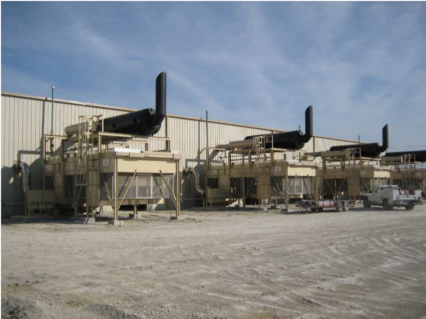
Enclosed Compressor Unit Provides excellent sound abatement
